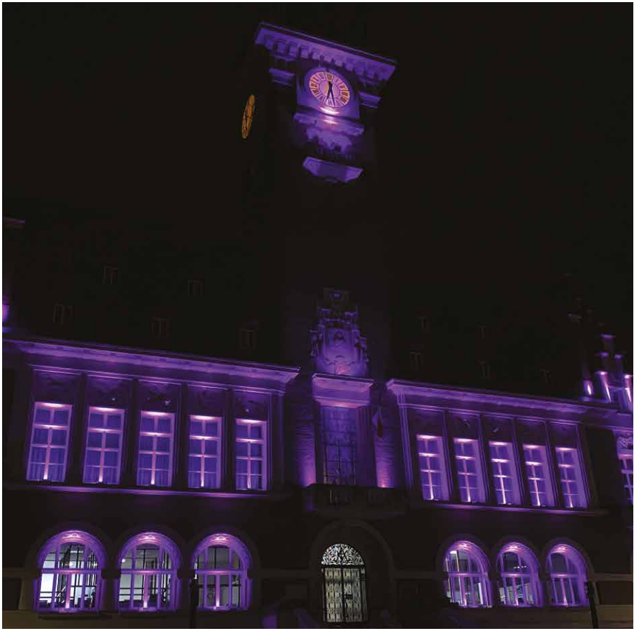
Architectural lighting on the town hall Albert
