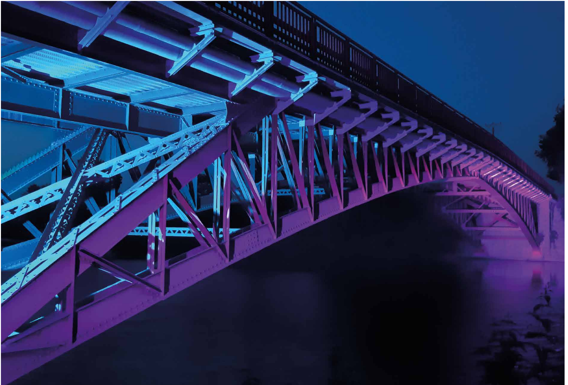
Architectural lighting on the Fillé-sur-Sarthe bridge Citizen Project
